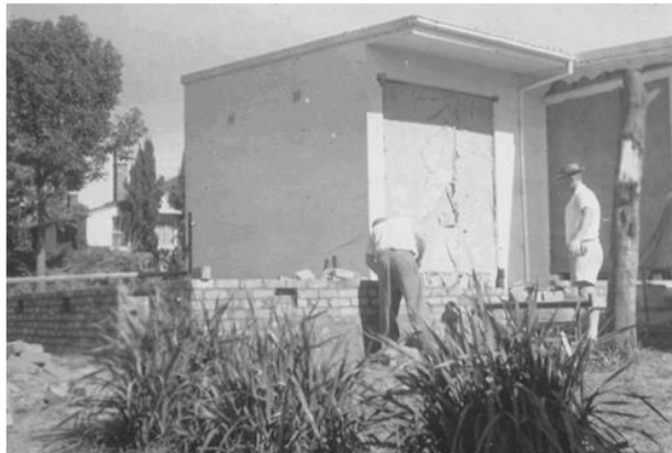
Figure 17: Lavery House second stage under construction, nd (c. 1955). Eastern addition to the house wing. Windows of the original Bedroom and the east end of the Living area have been removed for re-use and the openings boarded up. Note also that the Chinese Elm has been effectively removed by being cut down to about 3 metres above the ground. (Source: Lavery Family courtesy of Piers Lavery, October 2020)
