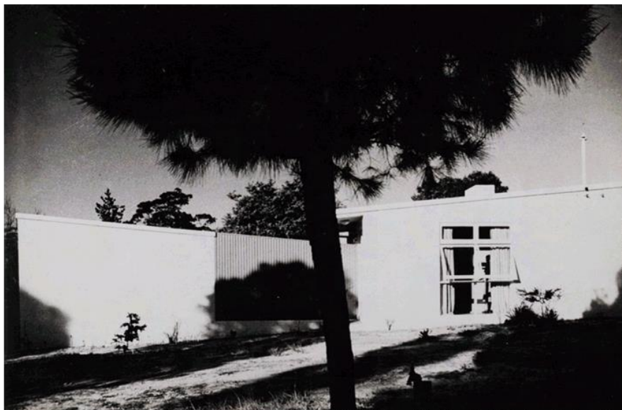
Figure 4: Lavery House, Turramurra [sic – now known as Wahroonga], 1952 (Source Max Dupain). This is the original west (front) façade of the house before the additions of 1968. The timber screen wall was painted bright blue and gave privacy to the courtyard between the two buildings. (Source: C. Boesen, 1979, Sydney Anchor: A Profile , Volume 3 Plate 54)
